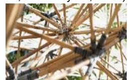
extremely light-weight and elastic. In this context, the students used this long-established material to create a pavilion weighing just 200 kg. Spreading in three directions to cover a total area of more than 40 m<sup>2</sup>, its minimal supports contribute to the etherealness of the structure. This design-to-fabrication process depends on digital technologies, using purpose-made digital design tools to generate this ultralight yet complex structure.
